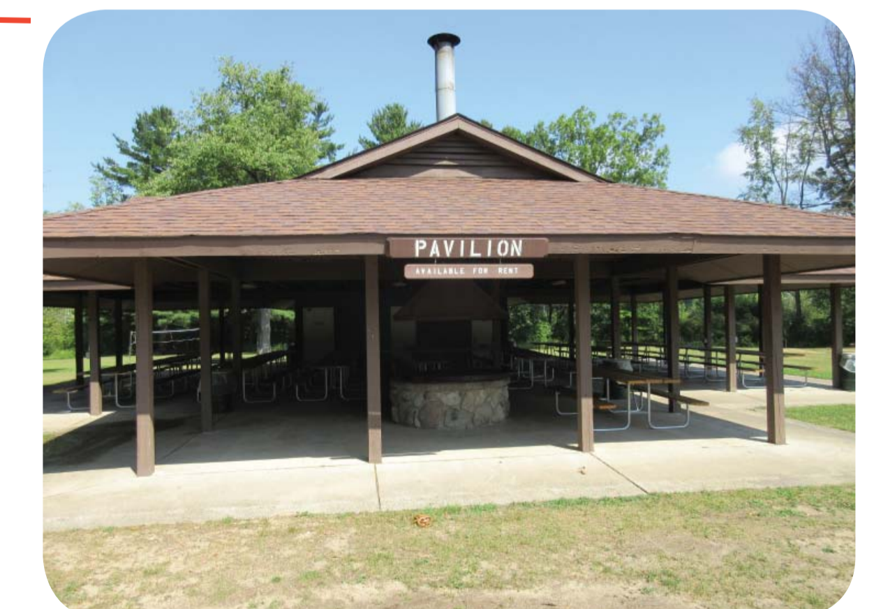
PICNIC SHELTER AND PAVILLION WITH RESTROOMS.
